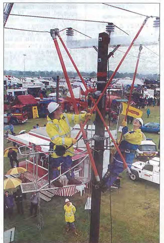
Manweb Linesmen show how to change an insulator with the line still live – just one of the demonstrations at the Cheshire Show.
